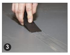
Using the Rapid Floor Seam Finishing Tool, immediately pull across the uncured weld at 20° angle with the bevel facing down. Focus pressure 1″ from the end of the finishing tool to leave a thin transparent film on the tape.
