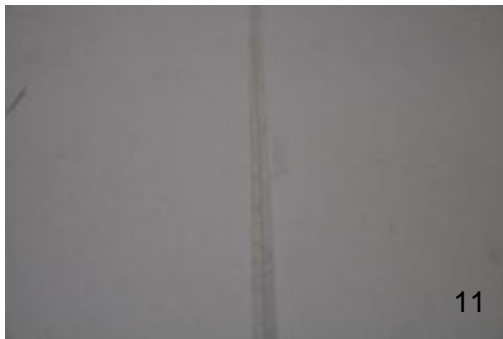
11. Finish groove seam.
