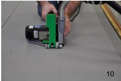
10. Power groove seam 3/16" deep.
