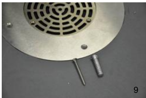
9. Secure drain ring to substrate. Only use #10 2 ½" stainless steel screws (tapered head) with lead anchors.
