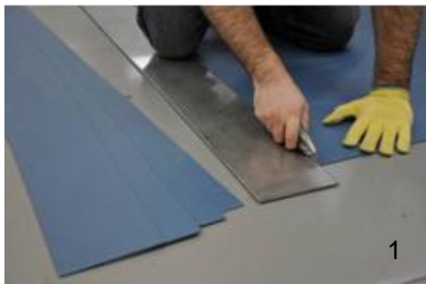
1. Use a 5’ x 8’ sheet, cut into 6” x 8’ strips to create 80 lineal feet of cove base
