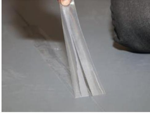
**Image 11:** Remove tape immediately after smoothing
