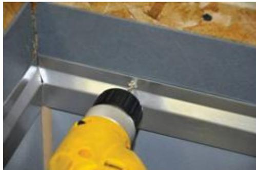
**Image 27:** Pre-drill using 1/8” drill bit. Use screws and anchors appropriate for wall type.
