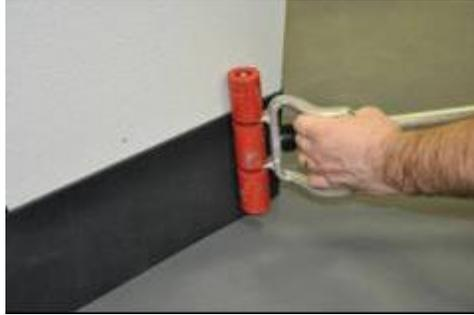
**Image 20:** Immediately hand-roll or rubber hammer to set into cove base tape or adhesive
