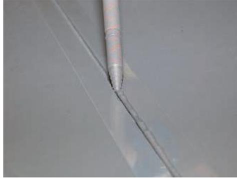
**Image 9:** Dispense Protect-All Rapid Weld into taped seam.
