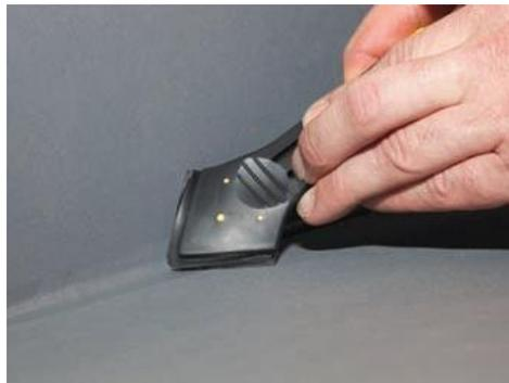
**Image 23:** Smoothing seam with Radius Finishing Tool
