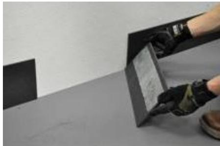
**Image 19:** Adhere using a 3" or 4" band of web-reinforced, acrylic 2-sided tape
