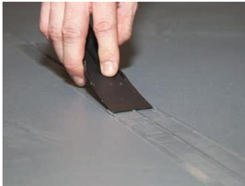
**Image 10:** Smooth seam by maintaining 20° angle in one pass.
