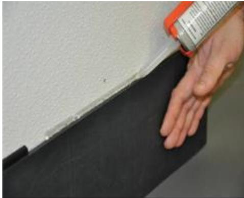
**Image 25:** Seal the top of the cove base with a continuous bead of sealant.
