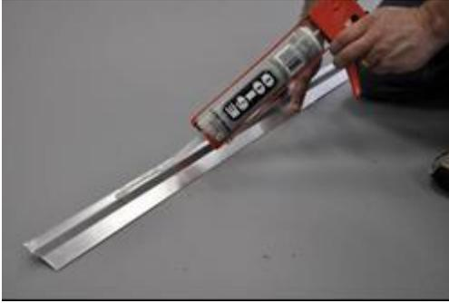
**Image 26:** Seal back of cove cap (aluminum or stainless steel) with E6100 before securing to wall.
