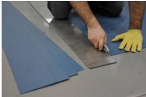
**Image 16:** Use 5'x 8' sheet, cut into 6" x 8' strips
