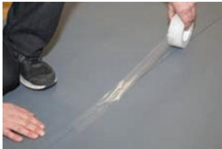
**Image 2:** Protect-All Rapid Weld Seam Tape over groove
