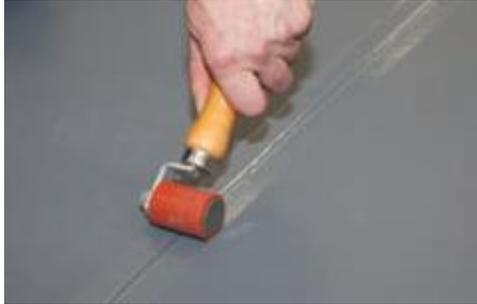
**Image 4:** Seal the Protect-All Rapid Weld Seam Tape
